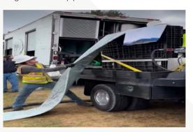
Sometimes it is necessary to assist or pull liner slack from the refrigerated truck or the end of a wet-out platform into the pipe being rehabilitated. Using a spreader bar is a great option instead of pull ropes wrapped around the liner, or lifting straps that can crush the liner, displace resin and destroy fiber orientation with GRP products. A good quality control plan will result in the highest quality product and drive stakeholder confidence in pipeline rehabilitation.
