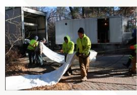
Liners delivered to the site in enclosed refrigerated trailers should also be set up in line with the pipe being rehabilitated. Pull in place or direct inversion methods should use roller bars or other devices to reduce stress and friction on the liner while positioning in place. Inspect the path the liner will traverse during installation,
