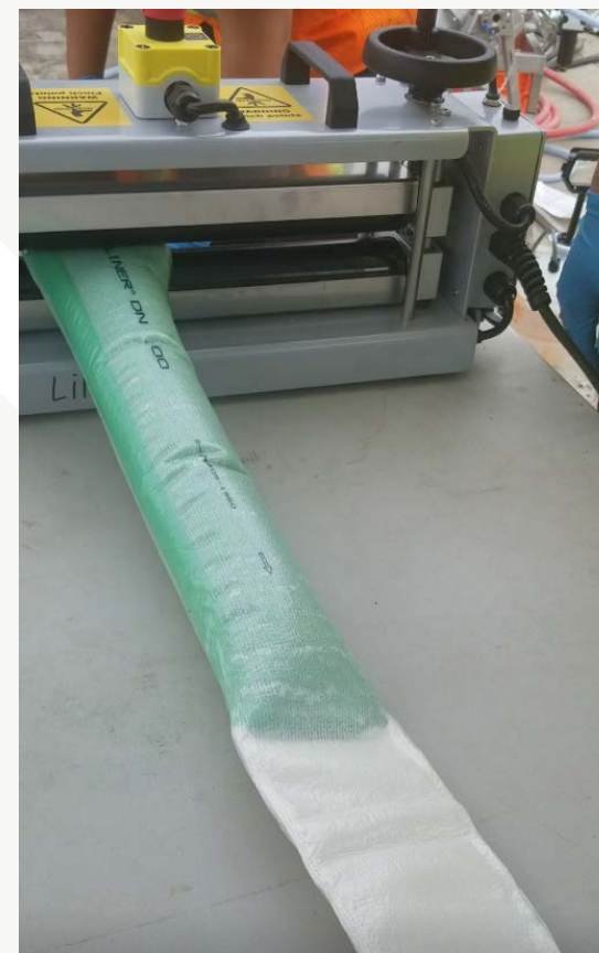
Wet-out liner before resin distribution and calibration
