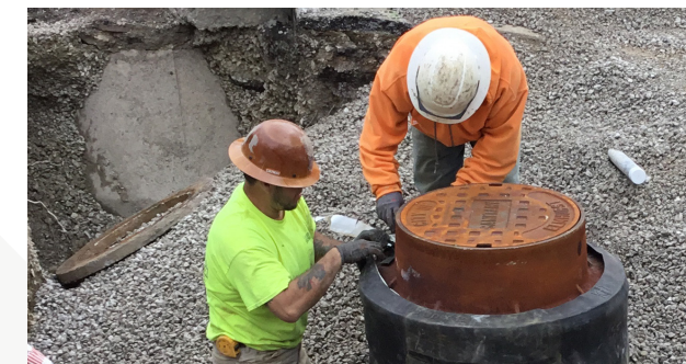
LEFT: Manhole vacuum testing. ABOVE: Manhole rehab.
