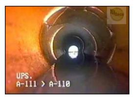
A BROKEN PIPE IS ONE IN WHICH PIECES ARE NOTICEABLY DISPLACED AND HAVE MOVED FROM THEIR ORIGINAL POSITION.
