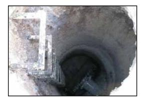
SEVERELY DETERIORATED, SEVEN YEAR OLD PUMP STATION DISCHARGE MANHOLE IN CENTRAL OHIO.
