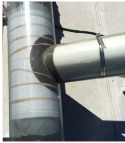
Typical lateral and main/lateral connection lining
