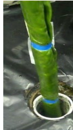
Folded liner pulled into cleanout
