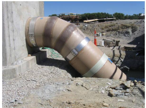
Above: Fiberglass fittings can be constructed in almost any configuration and angle, pictured is a 45-degree elbow with stainless steel closures.
